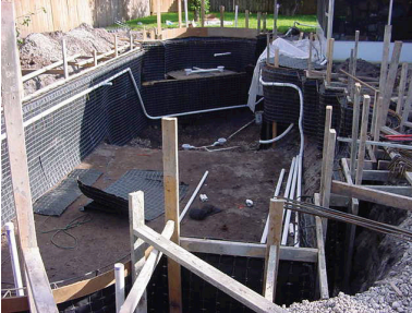
Shape of pool formed with rebar and wood braces
