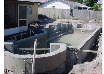
Ready for surfacing
