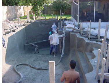
Fibercrete concrete sprayed onto rebar
